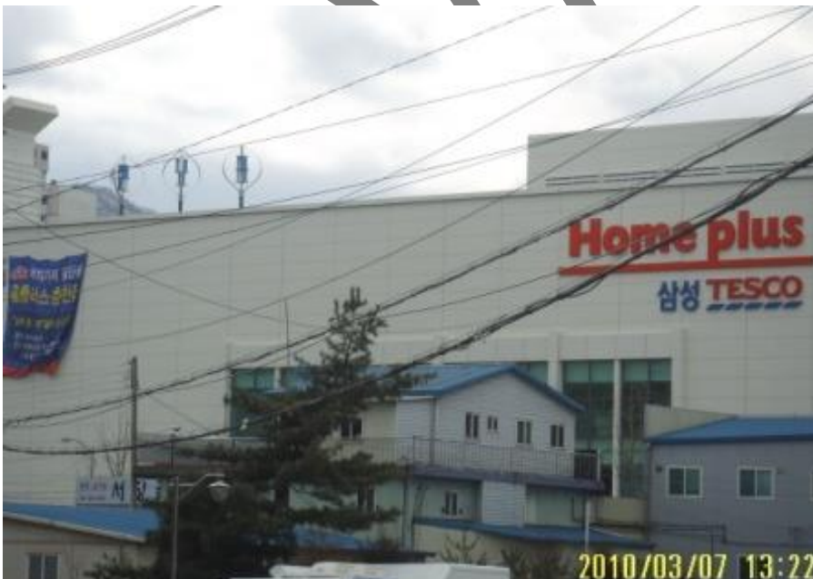
Rooftop application at a TESCO store, Korea
