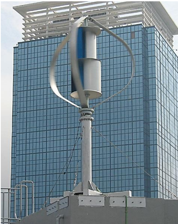
Rooftop application at EMSD building, Hongkong
