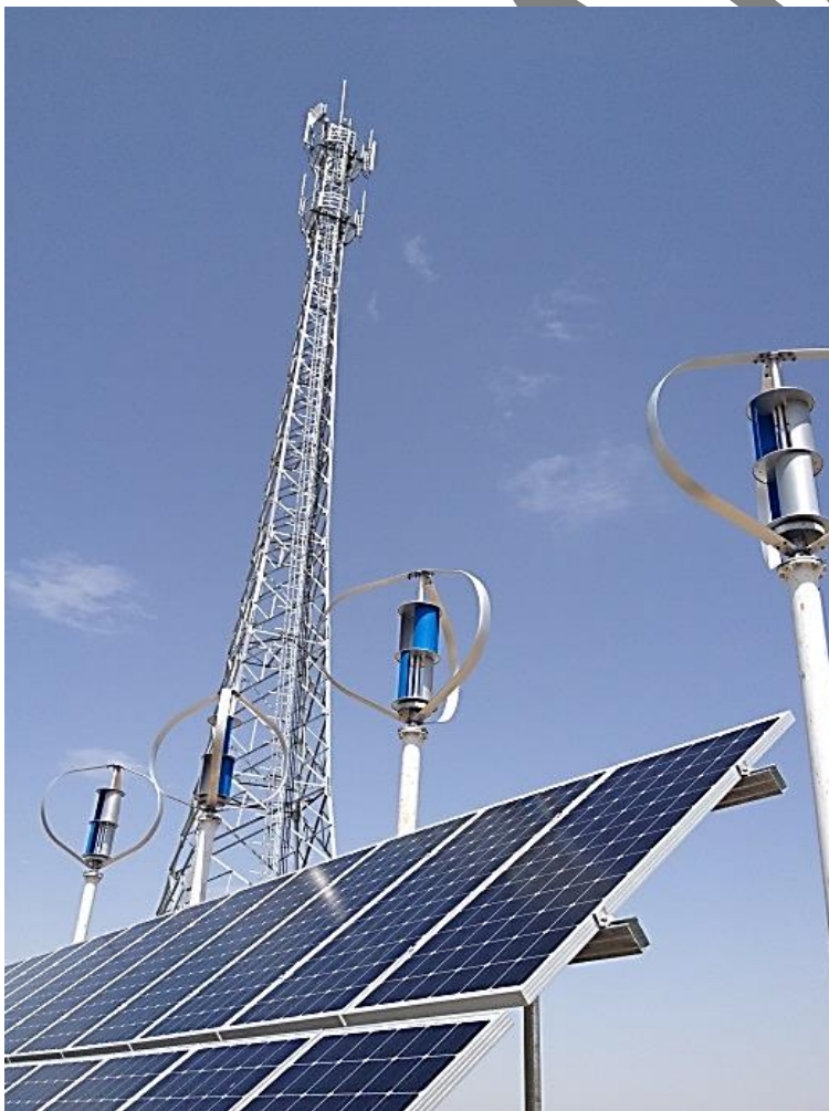
China Mobile telecommunication station, Xinjiang, China
