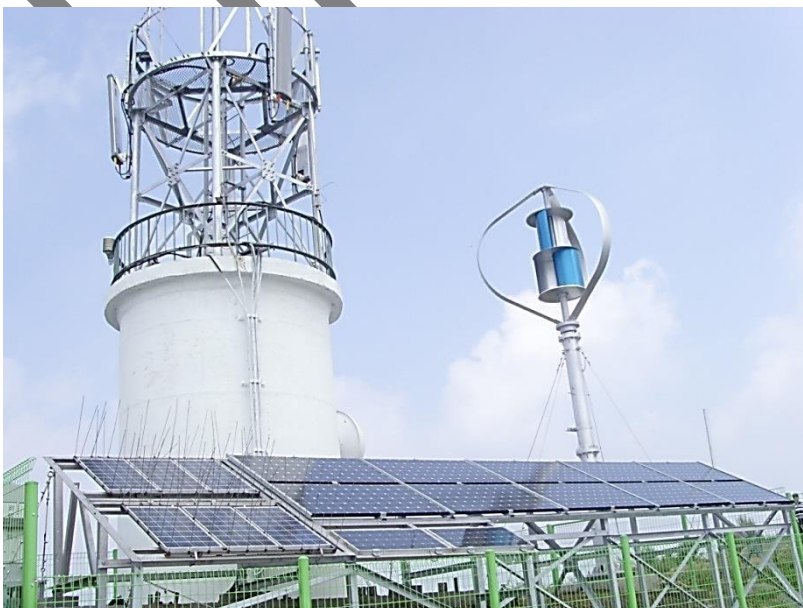
Telecommunication station, Korea
