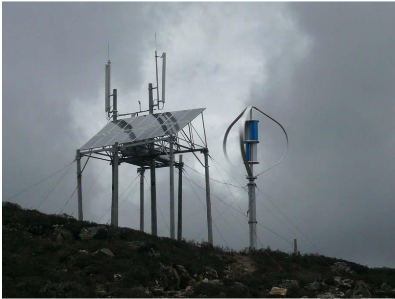
Telecommunication station, Tibet, China
